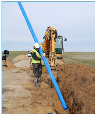
Correct ways of handling and transporting pipes
