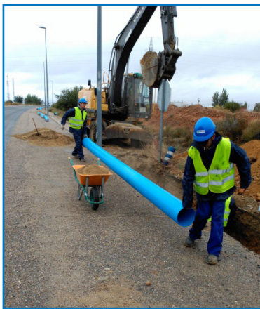
Correct ways of handling and transporting pipes
